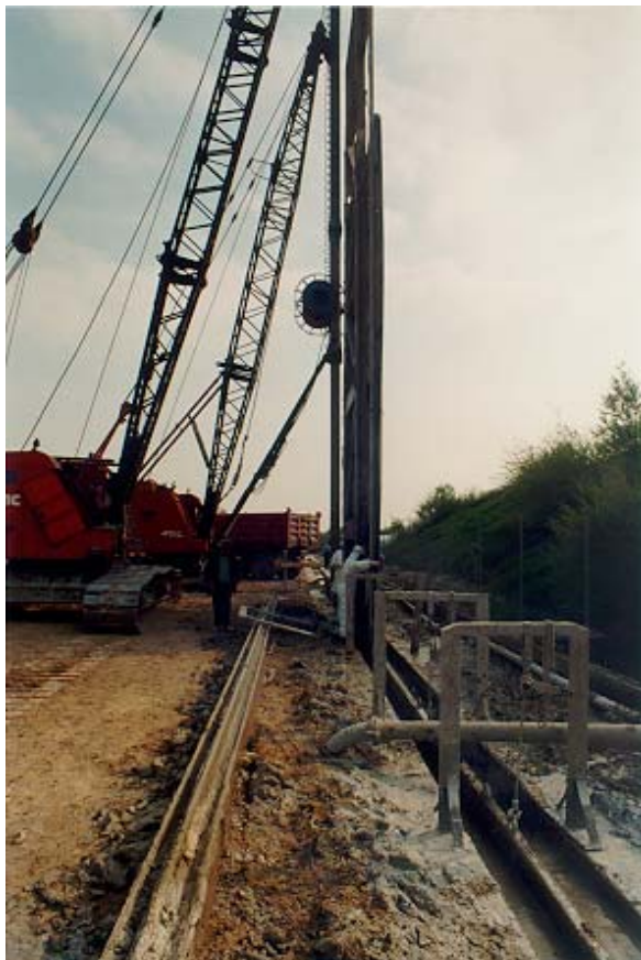
Downfeed of the AgruLock panels and subsequent hanging until the bentonite is cured
