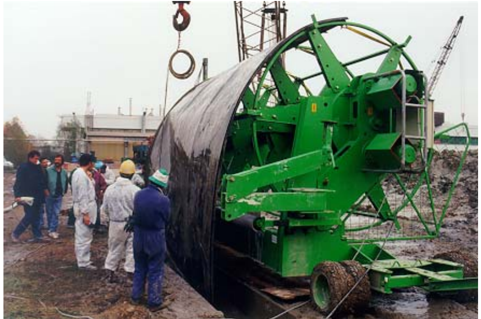
Lowering procedure with the drum
