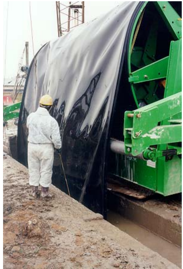
Downfeed of the panel using a drum with an electric drive unit
