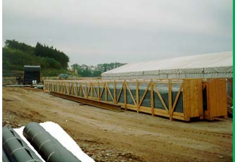
Storage of AgruLock profiles and AGRU HDPE liners in front of the welding tent
