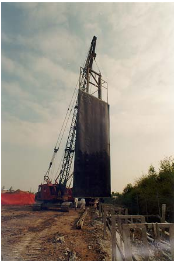
Raising the installation frame with the AgruLock panel attached
