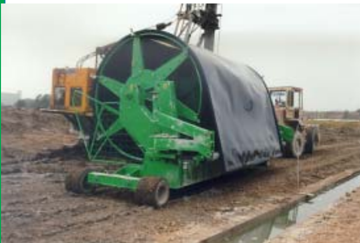
AGRU HDPE liner + 2 welded AgruLock profiles on the mobile drum
