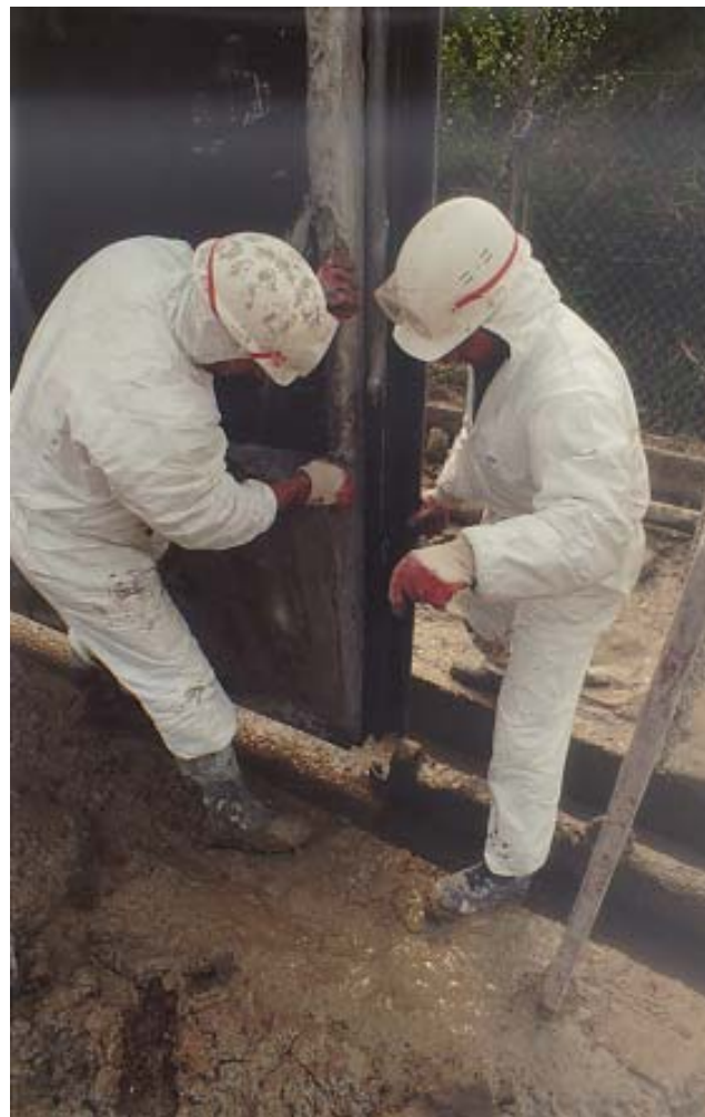
Insertion of the AgruLock panel into the profile already installed
